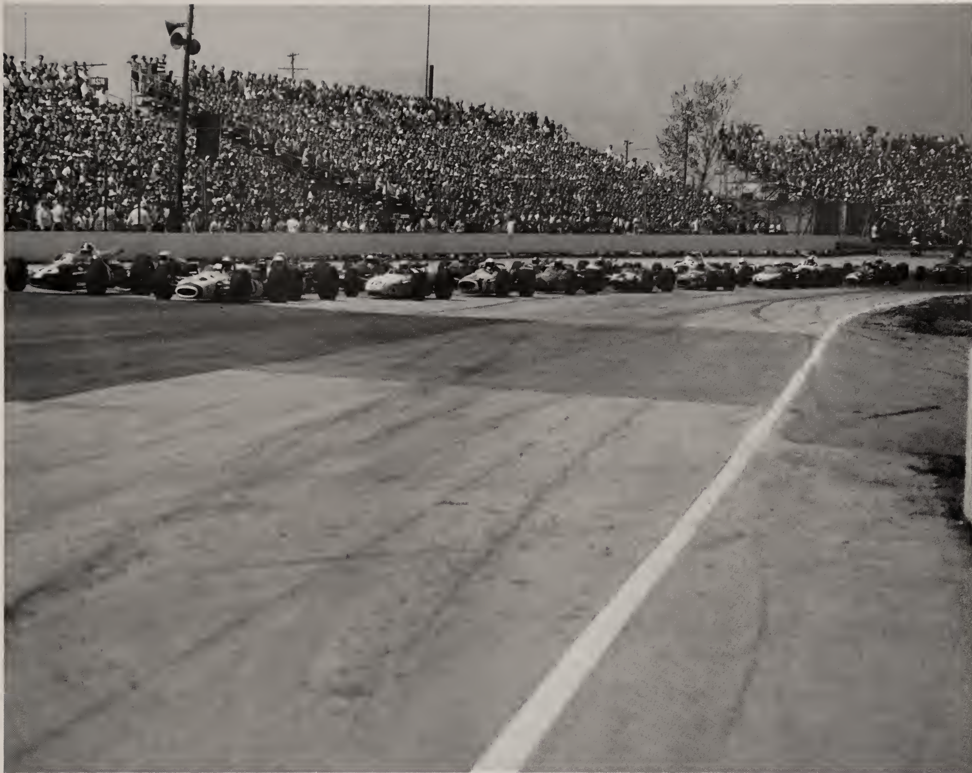
Details provided by this 1966 photo of Mario Andretti leading the pack to the start show some room for improvements in safety. Note the telephone pole on the outside of the wall, the armco barrier in the background and the blunt end of the pit
